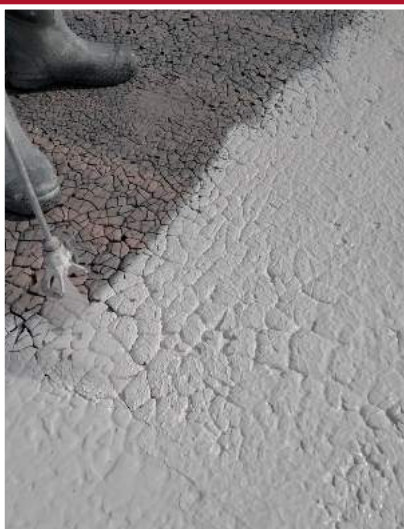
Making sure all cracks were filled.
