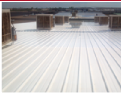
After: metal roof section.
