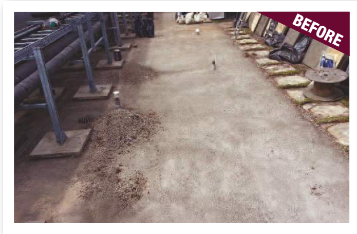
Scarborough Hospital, Asphalt Roof, Work begins
