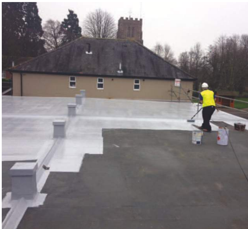
Seamless GacoPro being applied
