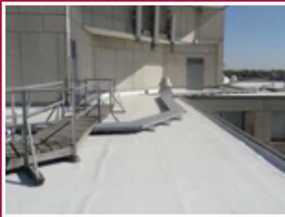
The completed roof coated with GacoFlex S20.
