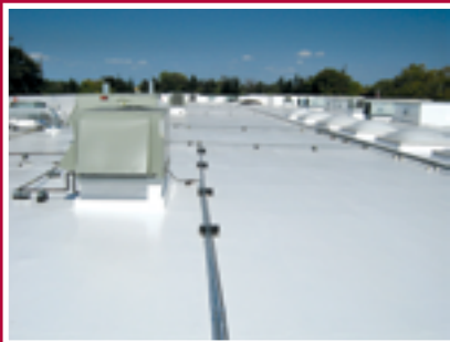
After applying GacoFlex S20 the roof surface is smooth and defect-free.
