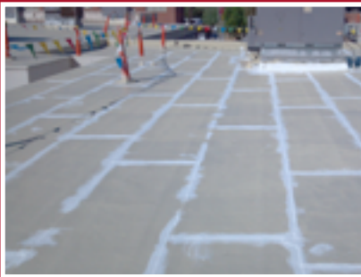
Before: built-up roof section.
