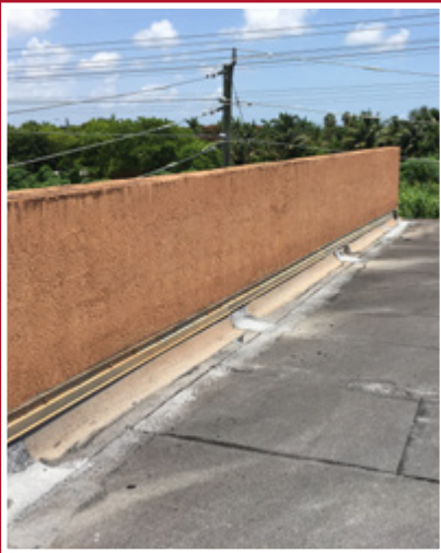
Before the roof restoration was complete.
