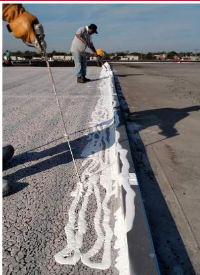
GacoFlex S20 being applied over GacoFlex E5320 2-Part Epoxy Primer/Filler.
